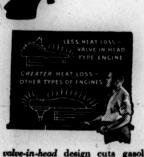
consumption still lower because there is less loss of heat through the walls of the combustion chamber in valve-in-head engines, and the advanced construction of the Chevrolet engine gives maximum heat (or power) saving.
