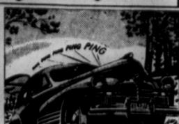
Engine knock or "ping", frequently caused by lower octane, war-time gasoline, can be corrected through motor tune-up, timing adjustment or—in serious cases—removal of cylinder head to clean out carbon.
