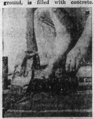
Greased form, set on leveled ground, is filled with concrete.
