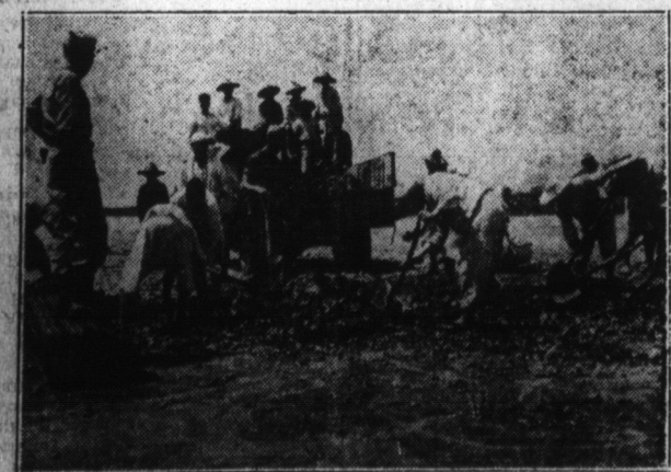
AVIATION ENGINEERS WORK KOREAN STYLE - Before adequate modern equipment was available, a small detachment of U. S. Army Aviation Engineers supervised Korean laborers in repairing this damaged runway. Supplies for the ground forces in the front lines were airlifted to this strip and then sent to their destination by truck and rail. Standing in the left foreground is Captain William Turner, in charge of the Engineers in this South Korean area, who directs tedious pick and shovel work.
