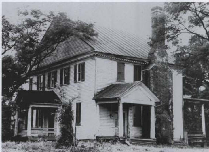
Western exposure of Cloverland, with side and rear porches and the massive brick chimney. (Courtesy of Karee Miller).
