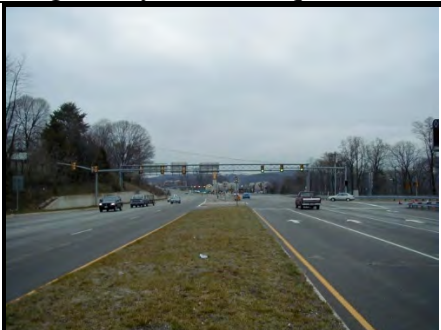
Gordon Boulevard, looking north from I-95 Bridge
