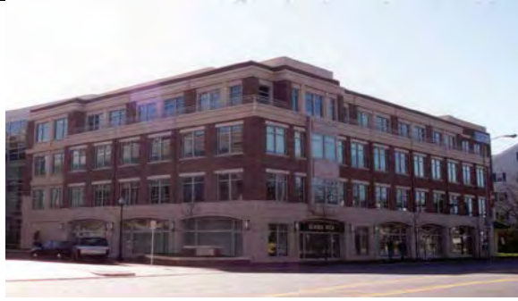
Good balance - Example of an asymmetrical façade that utilizes localized symmetry of window and ground level entranceways
