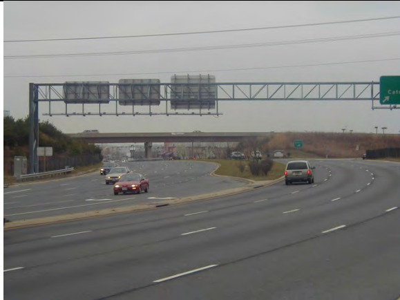
Prince William Parkway, looking west toward Horner Road Bridge
