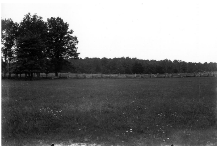
View southeast from near the viewshed point looking toward the Confederate position, 1896. Courtesy Dayton History
