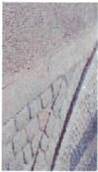
Crosswalk or Entry Apron surfaced in cobble or comparable special pavement material subject to County/VDOT approval.
