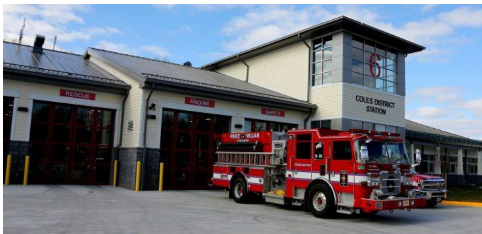
Coles District Fire and Rescue Station 6
