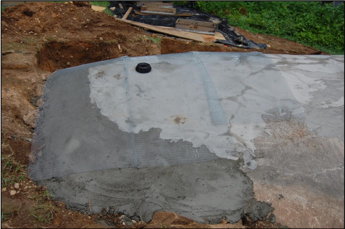
Plate 5-14. Application of Wire Mesh and Versa Bond Coats Complete
