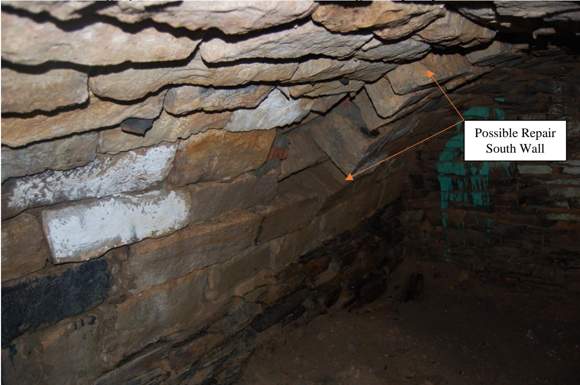
Plate 5-8. Photograph of South Interior Wall, Showing Likely Repair to Tomb's Arch
