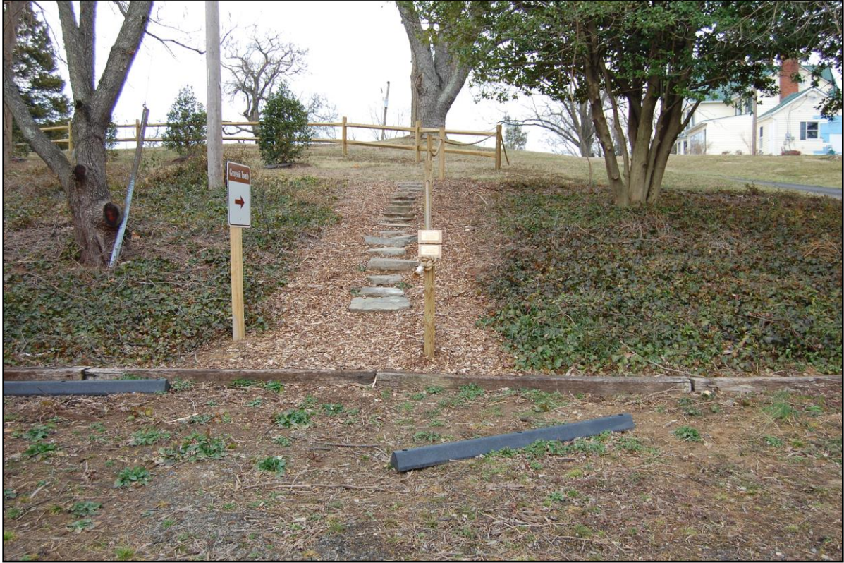
Plate 6-2. Parking Spaces and Trail Head Built, facing east
