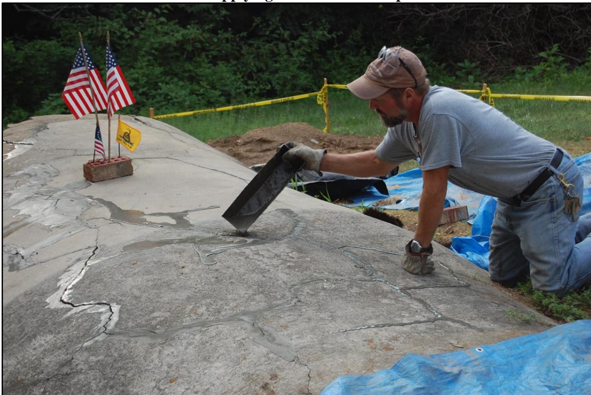
Plate 5-10. Fritz Korzendorfer Applying Versa Bond to Top Skim Coat
