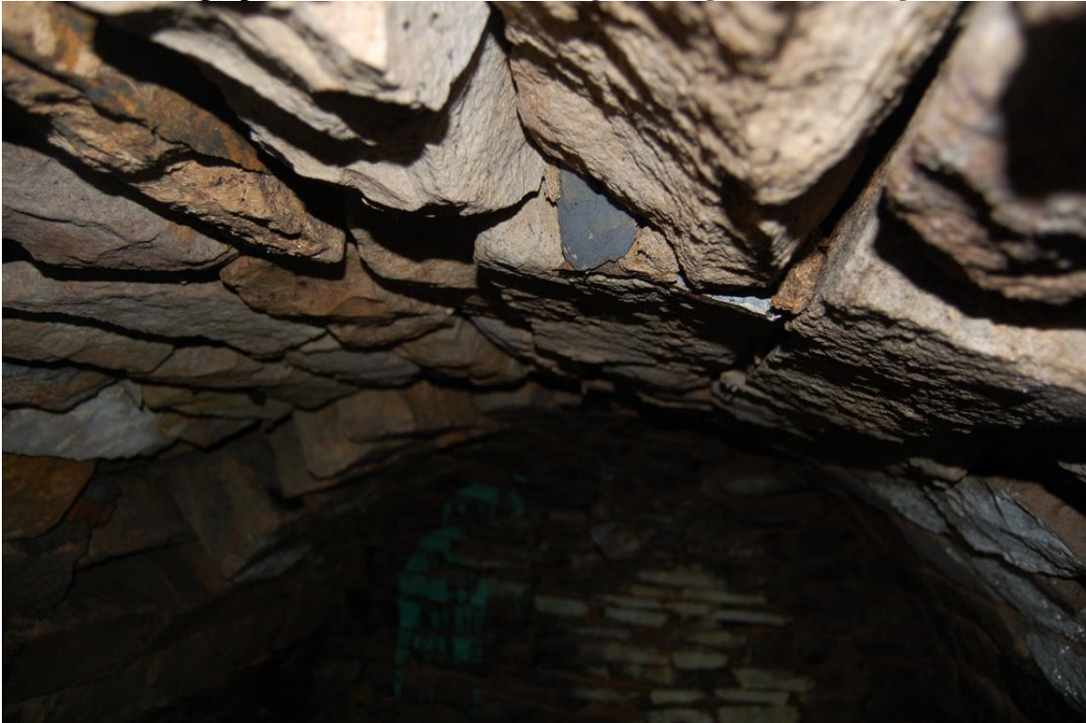
Plate 5-7. Photograph of Tomb's Arched Ceiling Showing Slate Chinking
