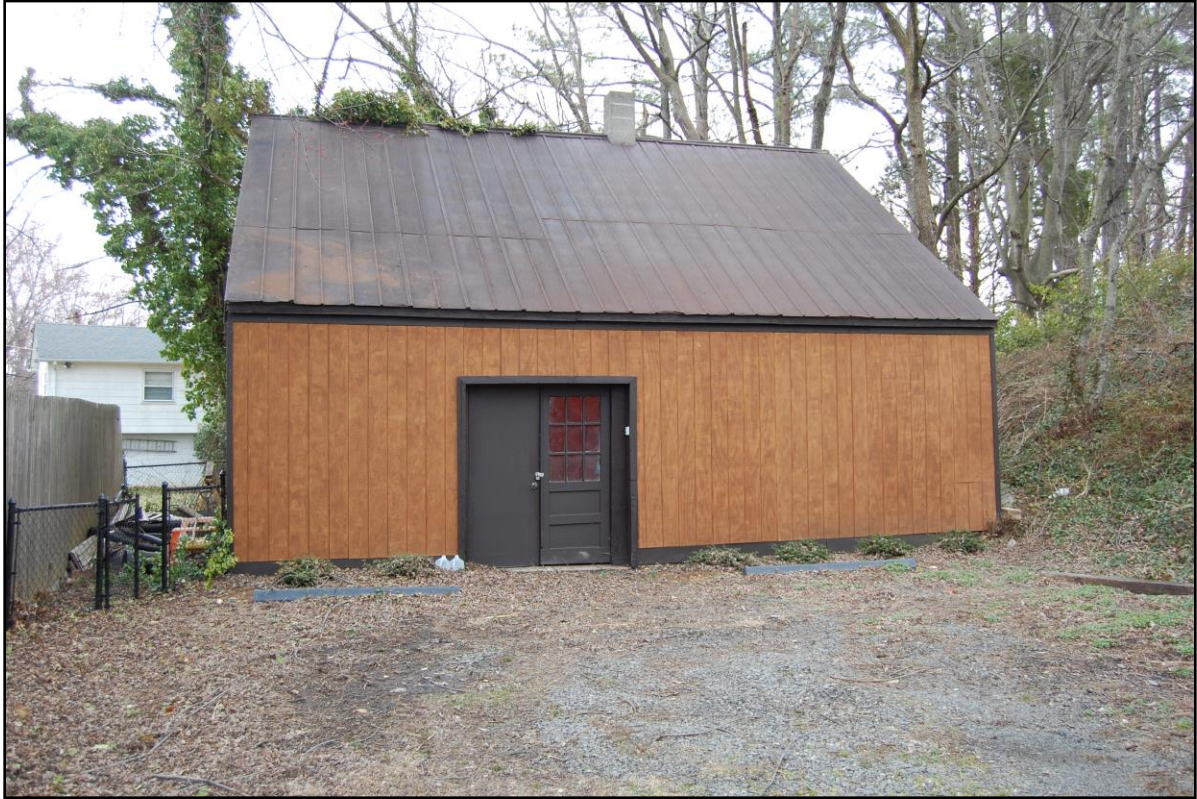
Plate 6-3. Refurbished Garage, facing north
