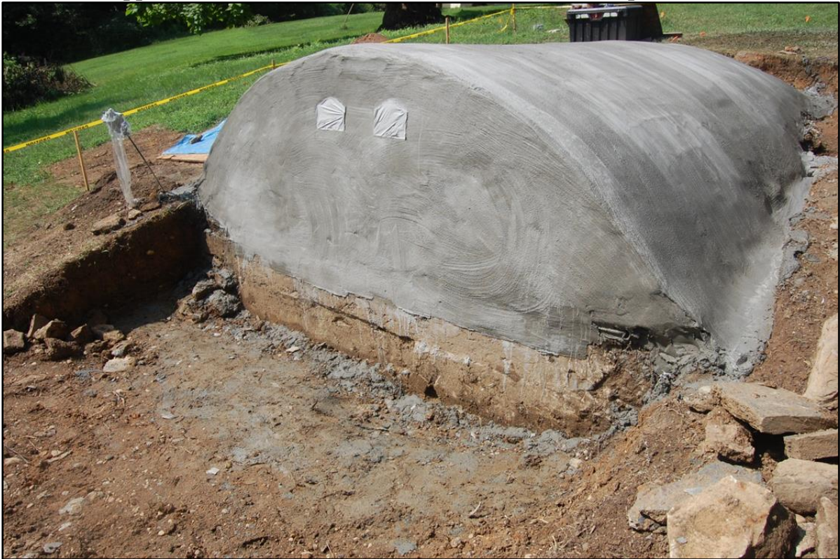
Plate 5-14. Application of Wire Mesh and Versa Bond Coats Complete
