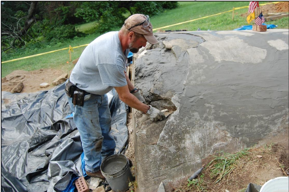
Plate 5-12. Fritz Korzendorfer Installing Galvanized Wire Mesh Reinforcing Tomb's Arch
