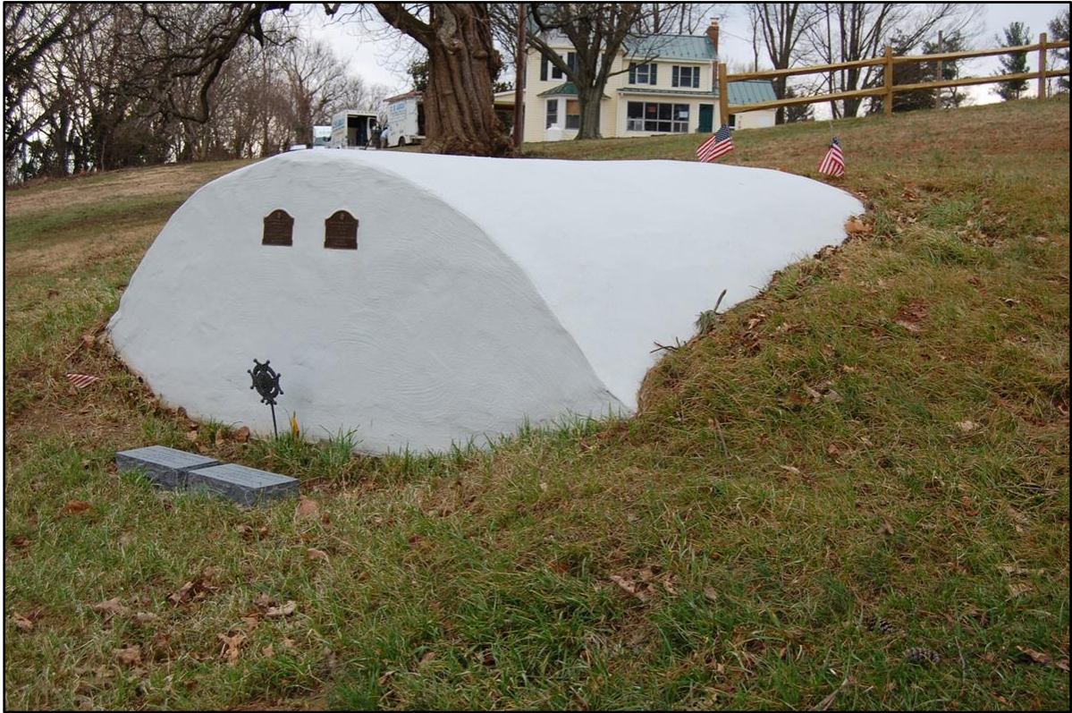
Plate 5-15. Project Complete with Application of Drylock® Waterproofer
