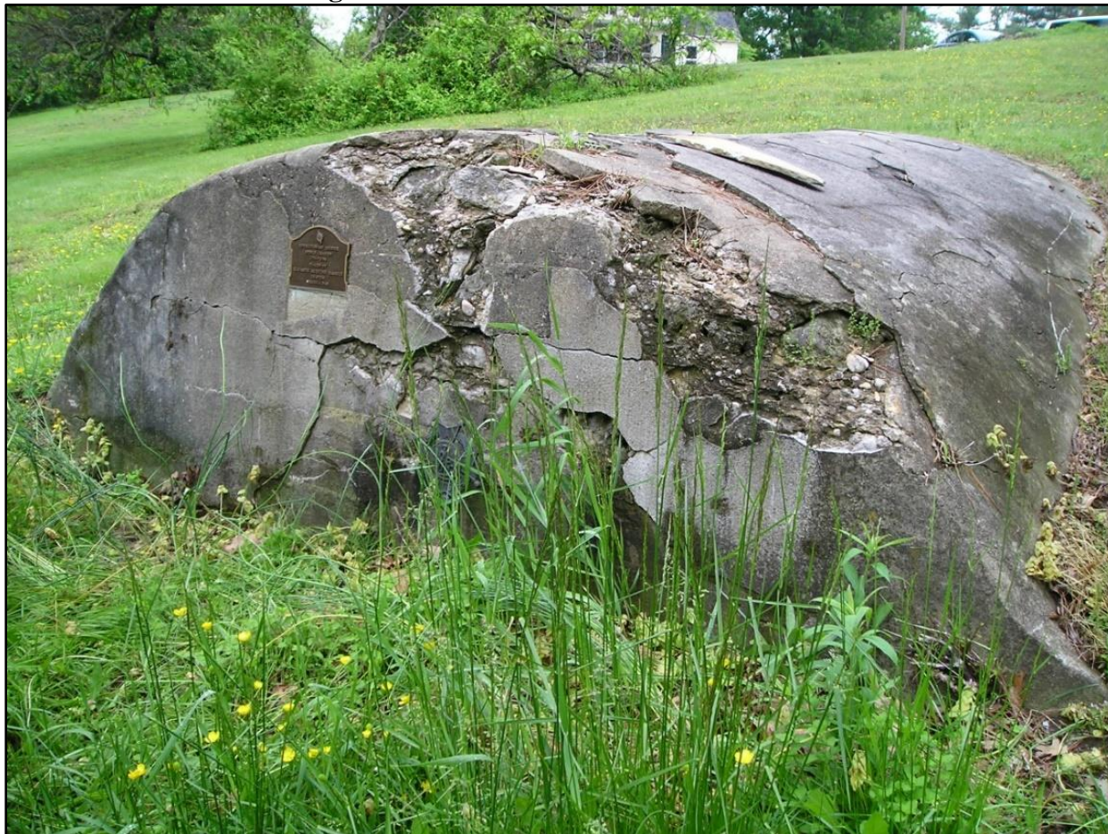
Plate 3-1. 2013 Facing Southwest at the East Face of the Tomb. Notice extensive spalling of skim coats and holes through the Tomb
