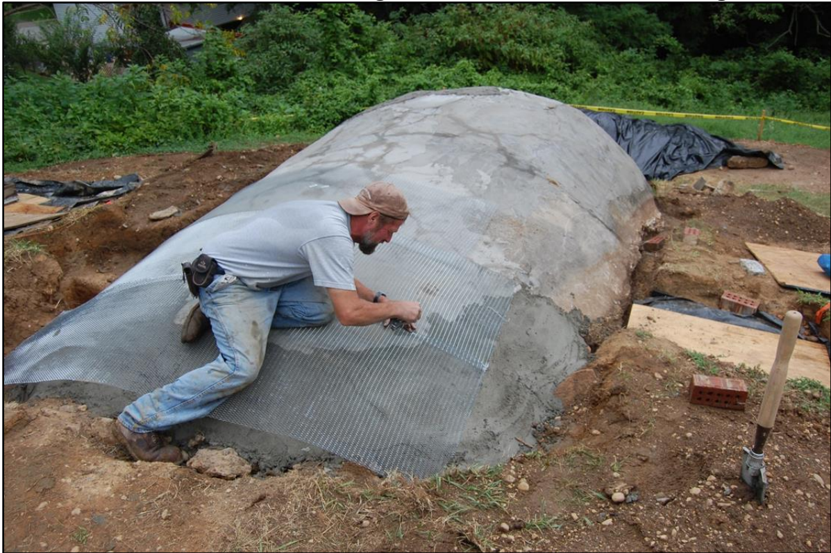
Plate 5-12. Fritz Korzendorfer Installing Galvanized Wire Mesh Reinforcing Tomb's Arch
