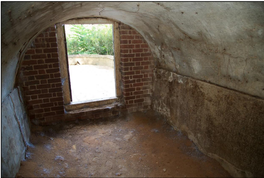
Plate 3-3. The interior of the Old Tomb at Mount Vernon. Photograph courtesy of the Mount Vernon Ladies' Association
