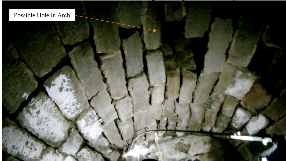
Plate 5-6. Video Still of Tomb's Arched Ceiling Showing Hole – Missing Stone
