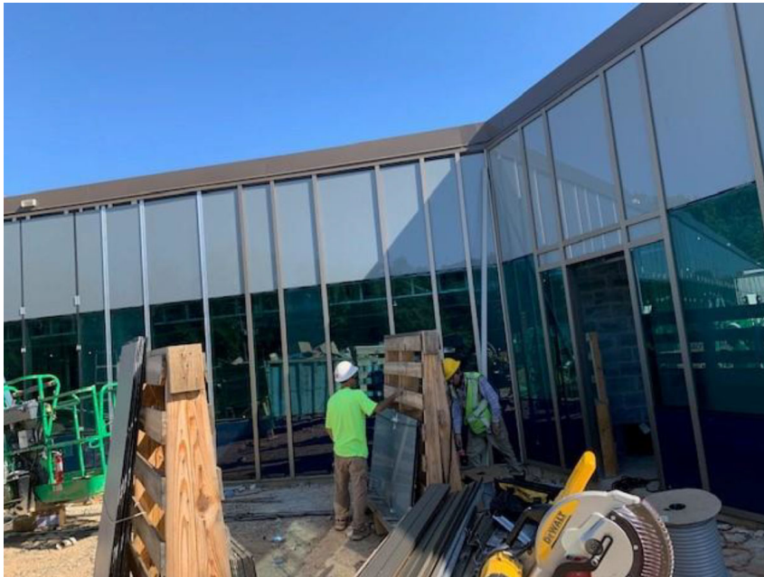
Installed curtain wall glass, clips, and caps
