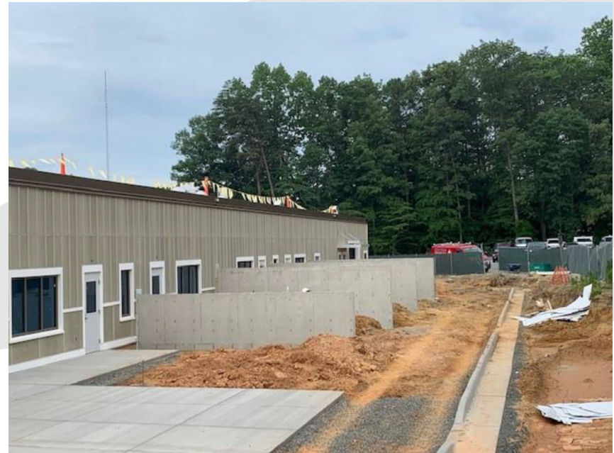
Exercise yard walls, curb, and site concrete
