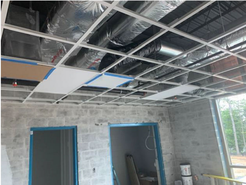
Ceiling grid and ductwork installed
