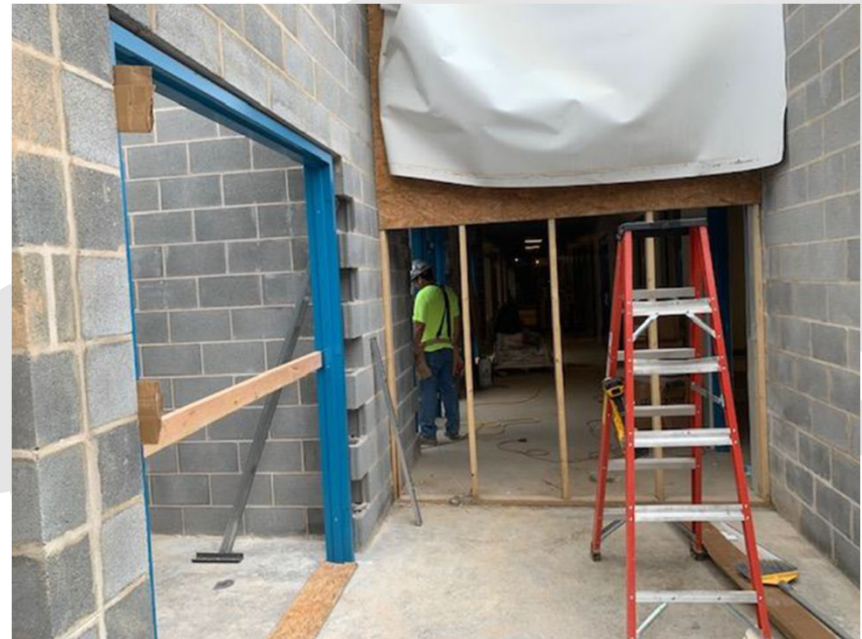
Installed interior door frames within restored space
