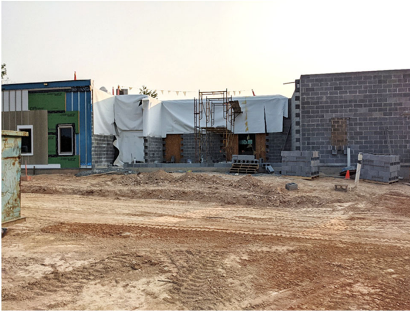
Constructing CMU walls for restored space
