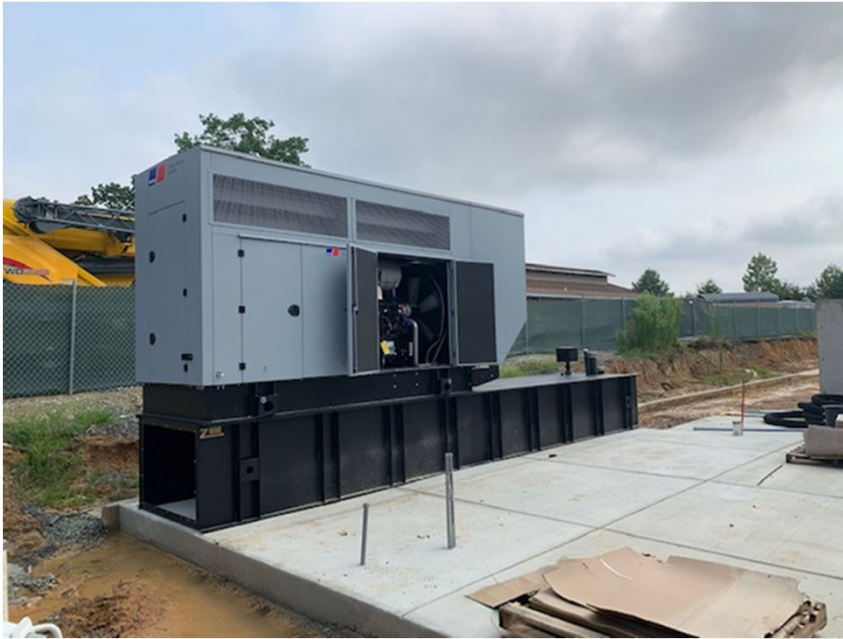
Set mechanical pad and generator
