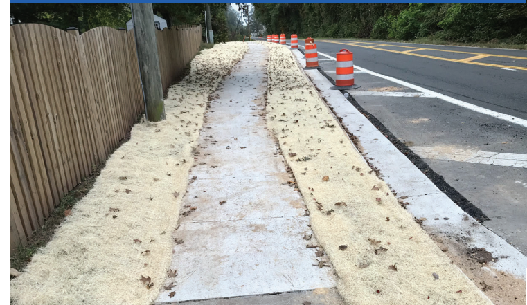
Lucasville Road Sidewalk
