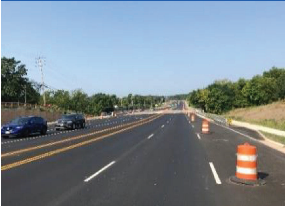
Route 28 Phase 3 - Linton Hall Road to Pennsylvania Avenue
