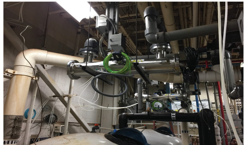
Chinn Aquatic Center – Ultraviolet Light System Replacement
