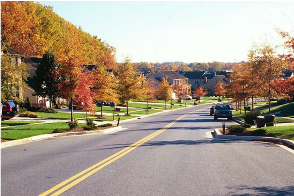
Figure 3.17.4. Choker in Suburban Residential Setting (Source: Scott Wainwright)
