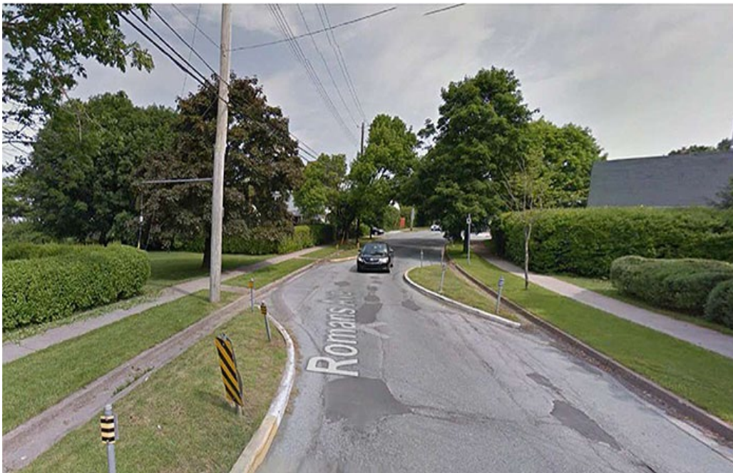
Figure 3.5.4. Chicane Designed to Retain Drainage Features (Source: Google Street View)
