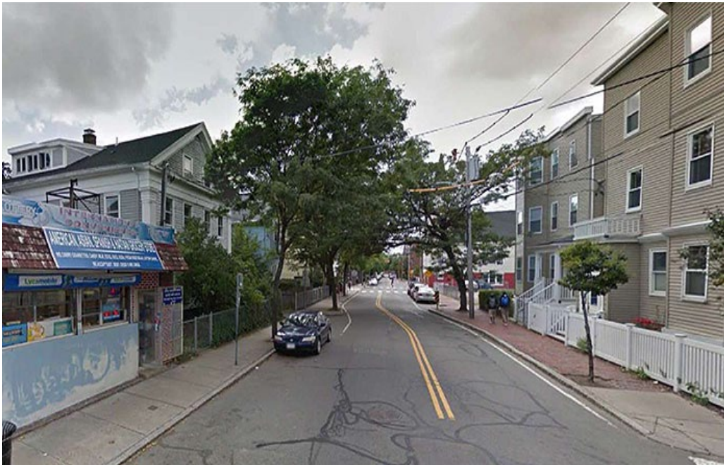
Figure 3.4.2. Lateral Shift with On-Street Parking (Source: Google Street View)
