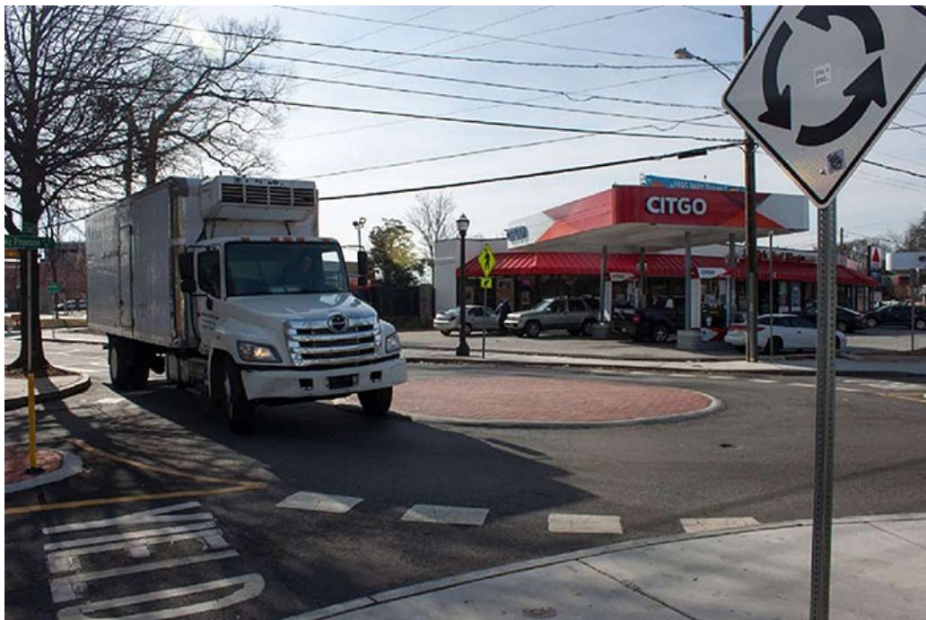
Figure 3.8.4. Mini-Roundabout with Truck (Source: Ian Lockwood)
