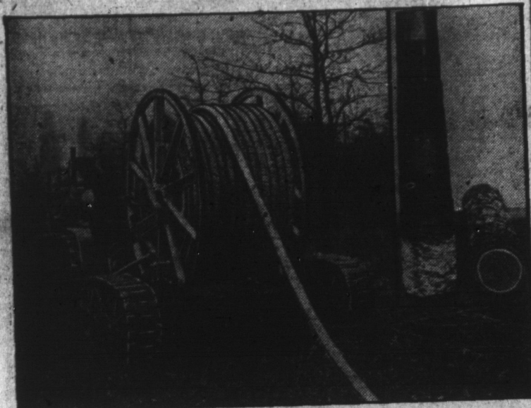
J. P. Ittner laying tape armored toll cable between Norfolk, Portsmouth and Suffolk, Va. This cable will be buried in a three-foot trench. Insert: Cross section of cable and method of protection.
