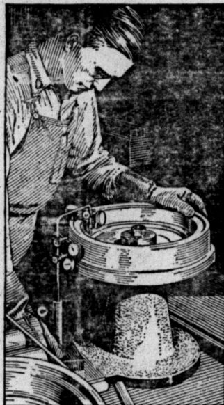
To achieve perfect fly-wheel balance, Chevrolet utilizes a special micrometer to hold every inch of the fly-wheel to uniform thickness.
