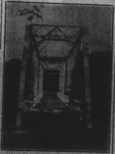
New Steel Bridge at Woodyard's Ford.
