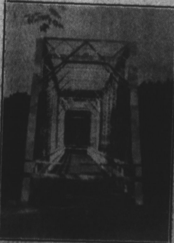
New Steel Bridge at Woodyard's Ford.
