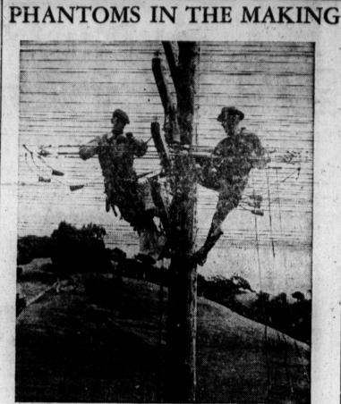
Phantoms-Telephone linemen transposing wires to provide phantom talking circuits.
