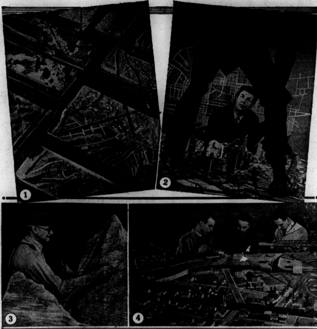
Above, craftsmen at work on world's largest animated scale-model to be feature of General Motors exhibit at New York World's Fair. (1) A few of the 408 panel sections which will be fitted together to create the completed "futurama"; (2) Norman Bel Geddes, designer of the model, inspects a detail of one of the cities; (3) here men are making mountains into molehills; (4) a trio of artisans lay out some of the half million houses and buildings designed for the spectacle.
