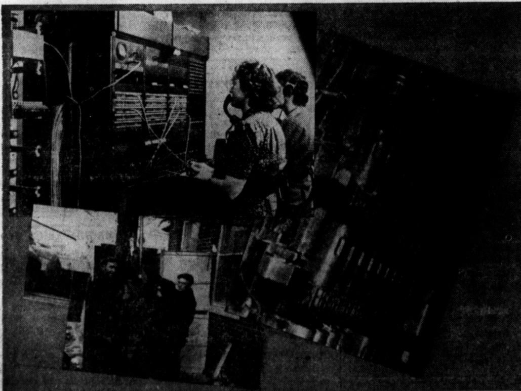
Views of the telephone system at Chatham where the central office was recently destroyed by fire. At right: the former central office; below: splicers at work connecting cables into the new office hastily established; and above: The temporary switchboard which was shipped from Kearny, New Jersey and cut in service a little over forty-eight hours after service was interrupted.
