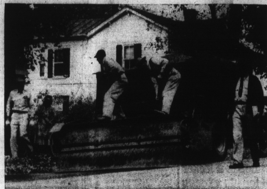
The State Highway Department is really spreading it on Manassas streets. Road crew is shown putting a top dressing of gravel and oil on West street.
