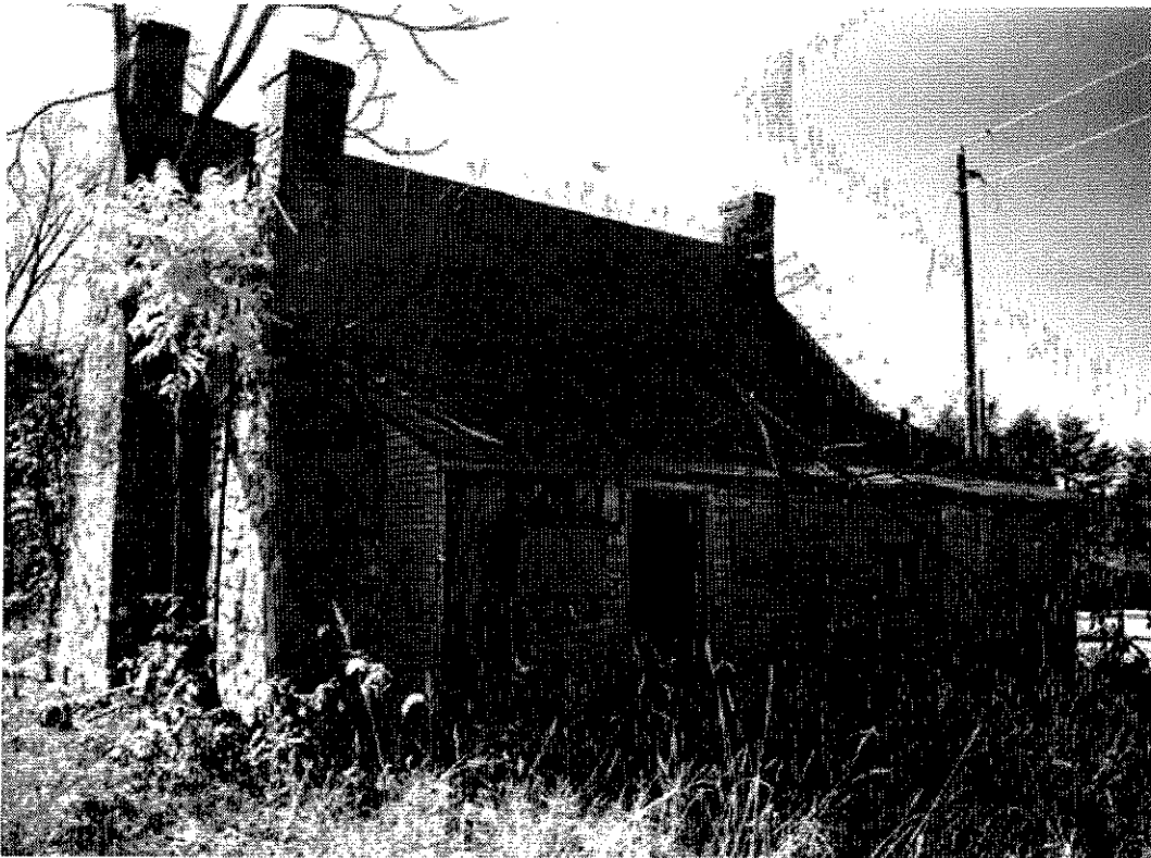
Figure 2: The Barnes House prior to the December 2003 move, showing the three chimneys
