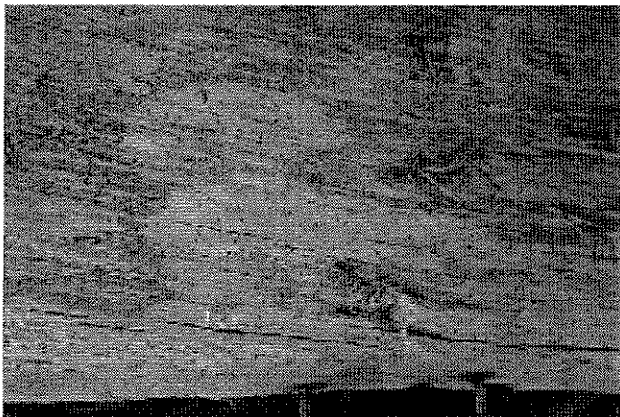
Figure 9: The joists, though similar in size, vary from hewn members to round "log" joists.
