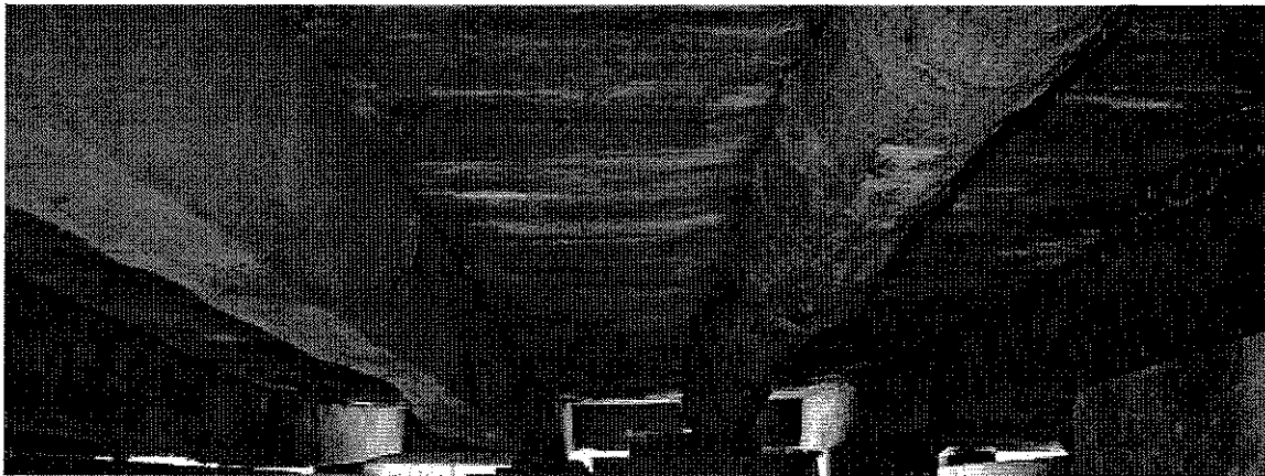
Figure 9: The joists, though similar in size, vary from hewn members to round "log" joists.
