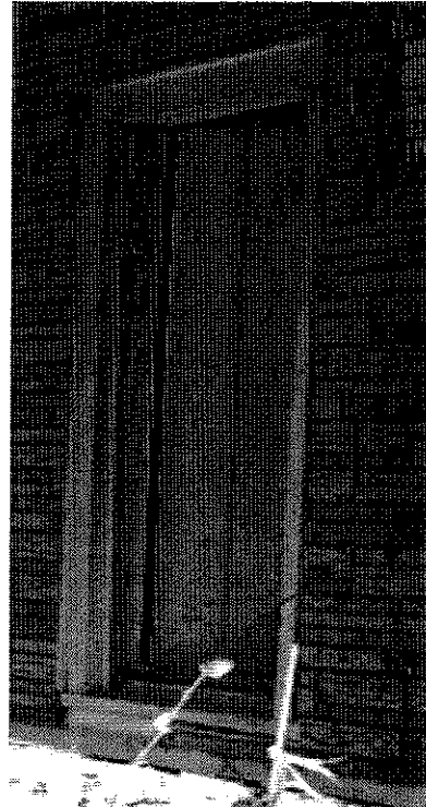
Figures 21 & 22: The plank doors at the front entrance and in the opening to the enclosed stair are excellent examples of the style and craftsmanship that accompanied the Tidewater frame tradition. They are constructed of beaded vertical boards with horizontal braces on the back. Fortunately, they are in good condition and can be repaired and retained. The house formerly had several others just like these two.
