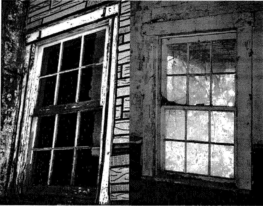
Figures 6 & 7: Exterior and Interior Views of typical 6/6 window sash, taken prior to the house
