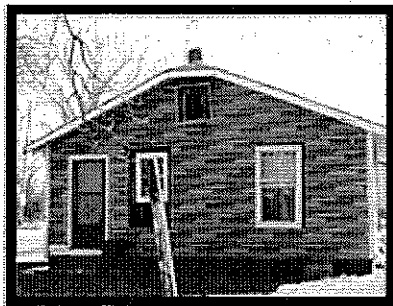
The popular 1950s look of cut sandstone could be achieved through the inexpensive application of Ranch Stone asphalt siding.
