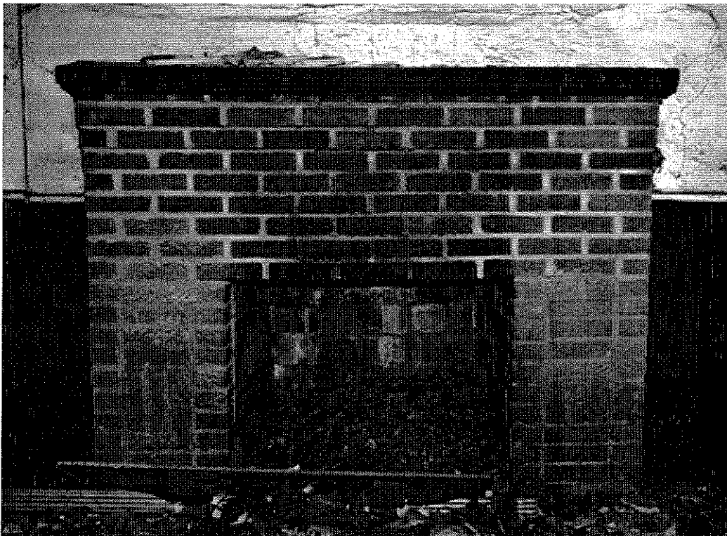
Figure 5: The brick mantelpiece (now gone) and knotty pine paneling dated from around 1960
