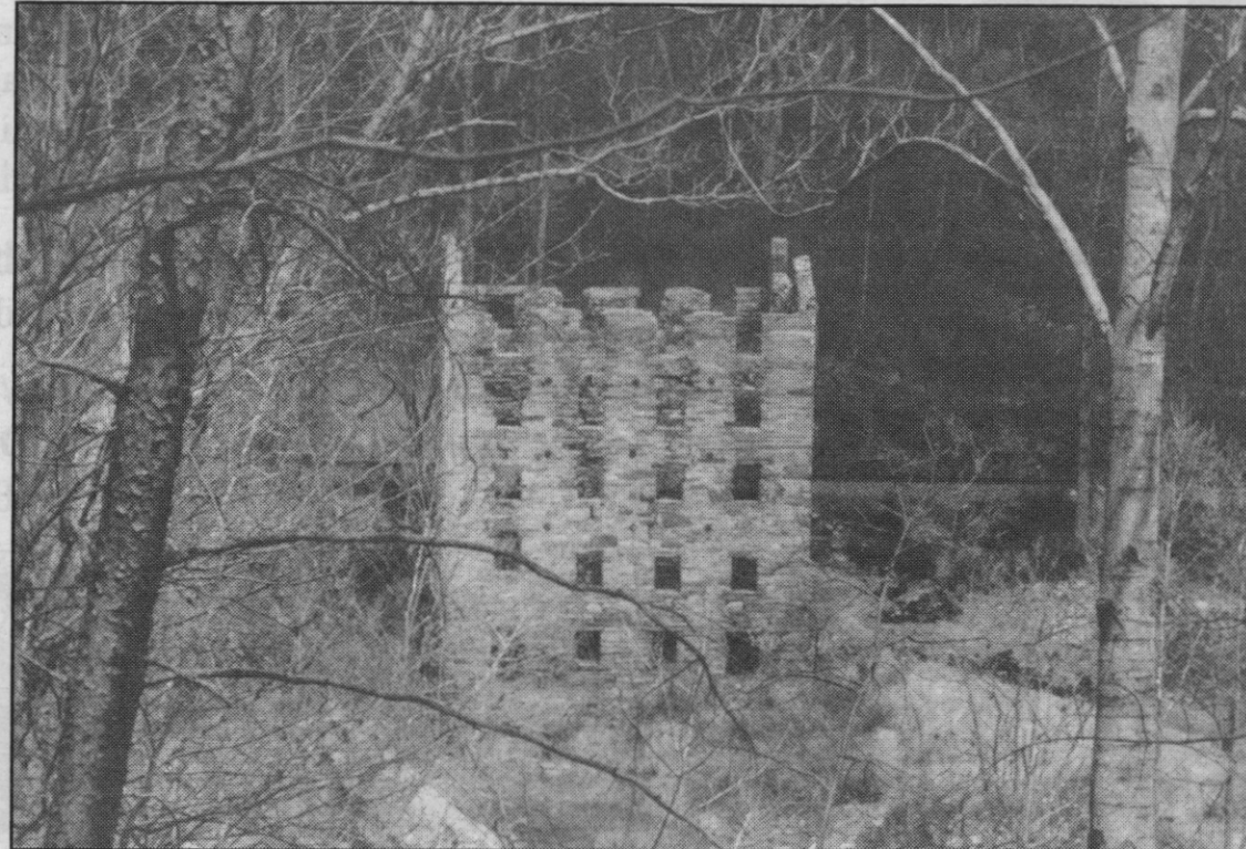
Beverley Mill soon after the fire of October 1998.
