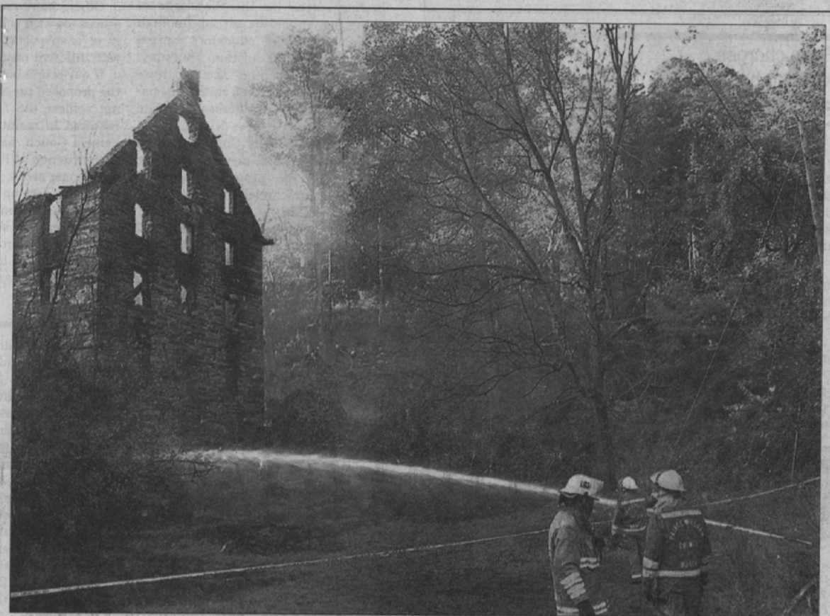
HISTORY GUTTED. Prince William County firefighters spray the smoldering Beverly Mill during a fire Thursday afternoon
