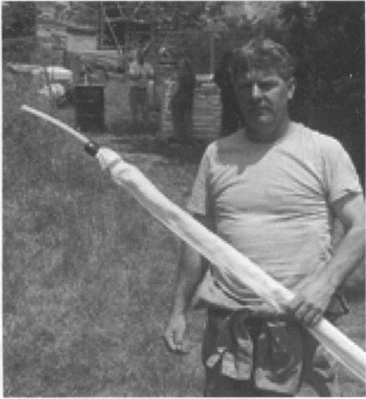
Anchor inserted into a "sock" ready to be inserted into a wall and filled with mortar.
