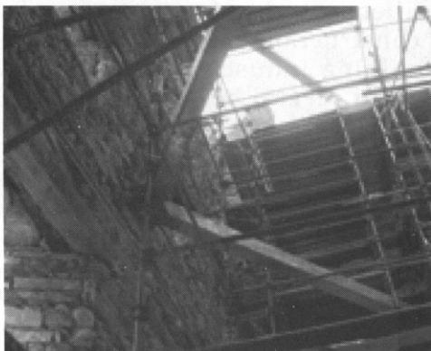
Installed steel beams.
