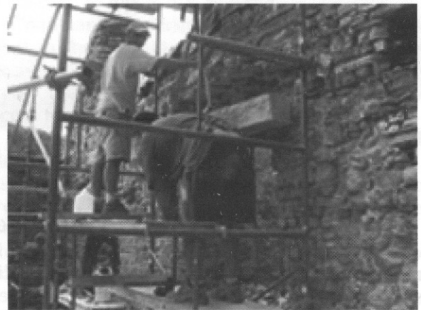
Installed stone lintel.
