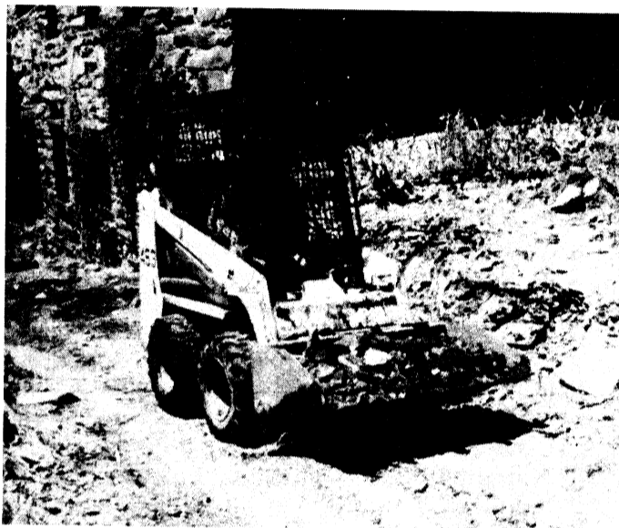
Bobcat Moving Debris at Beverley Mill - Photo by Harry Leach
