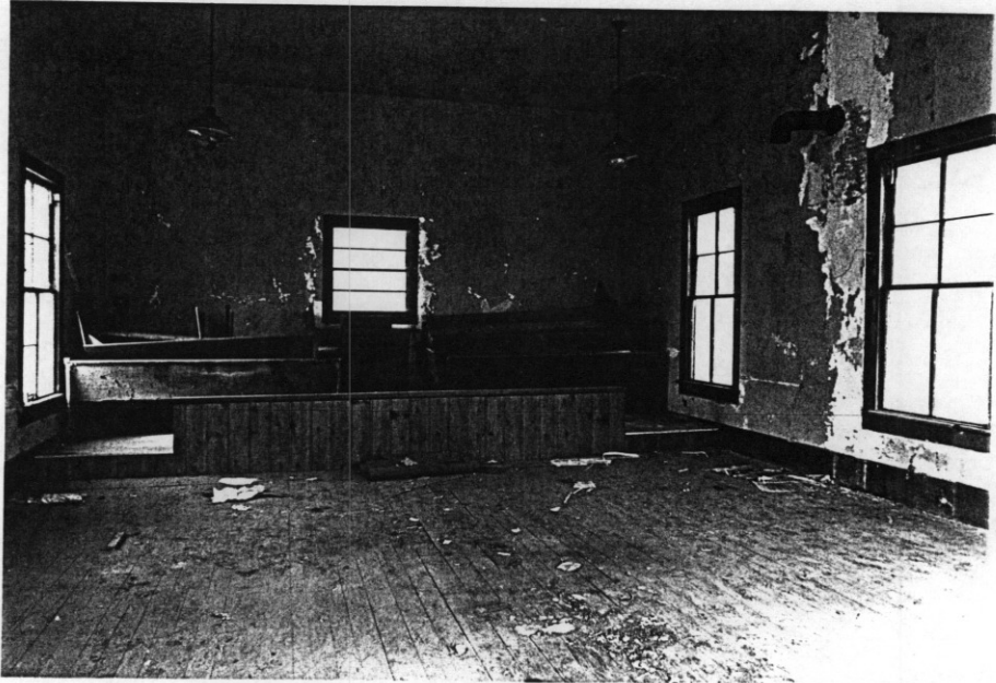
MAY 1980 REAR WALL (INTERIOR)
