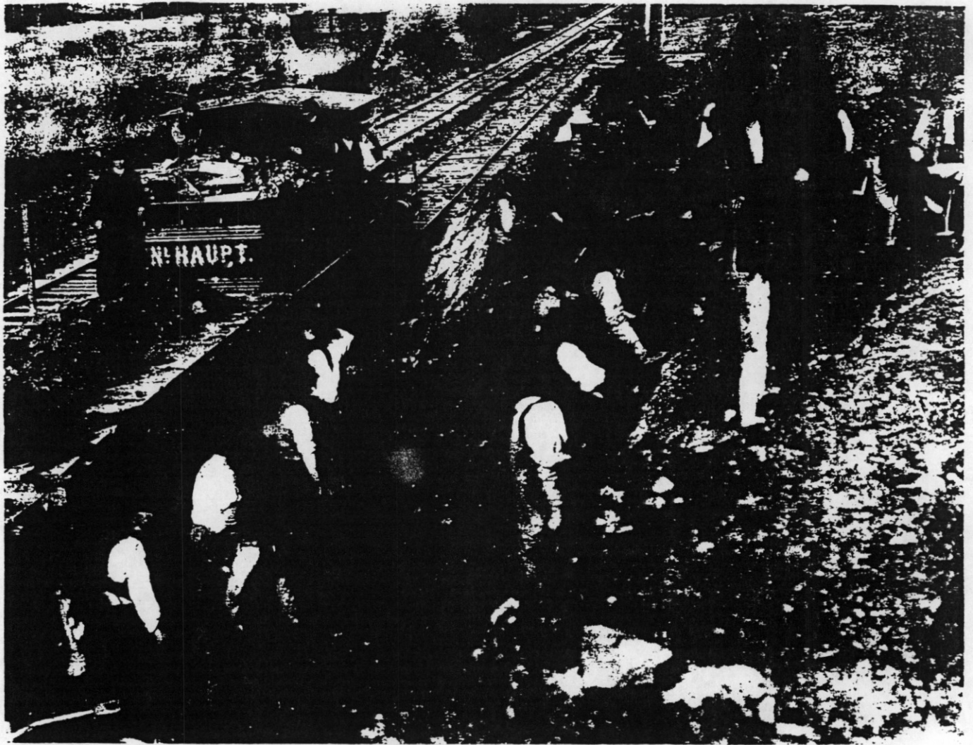
Workers repair the often-damaged Orange & Alexandria Railroad, a frequent target for raiders on both sides in the war. Warren was retreating up the railroad when Hill caught up with him.
