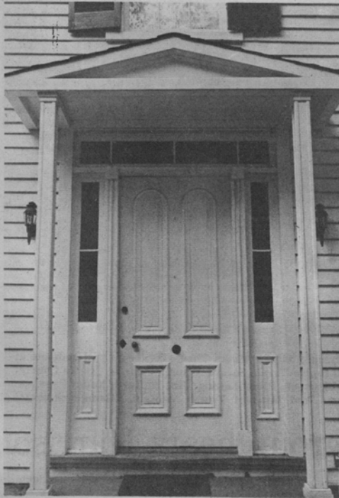
Just south of The Old Buckland Store on Mill Street, is another fine old place also restored by Mrs. Nathalie H. Roberts with an addition by Mr. and Mrs. Joe Campbell. It has been the home of two of Buckland's doctors: Dr. Kerfoot and Dr. Brown.
