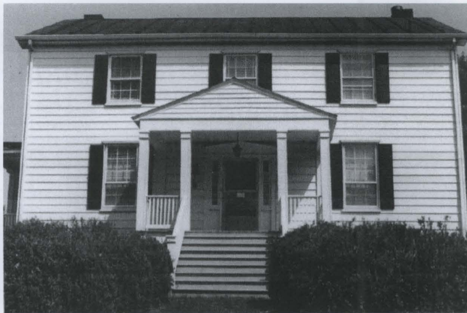
Burnside was photographed again in 1979 for a Virginia Historic Landmarks Commission survey. Alterations included aluminum siding, new porches, and extensive interior remodeling. Courtesy of RELIC.
