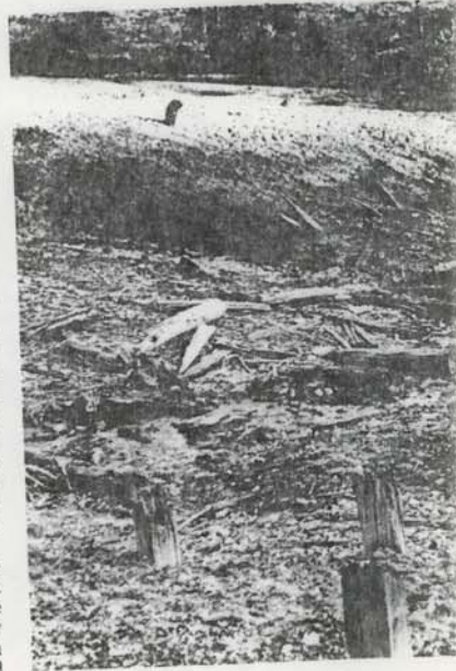
Ties mark path of railroad spur to entrance of old shaft
