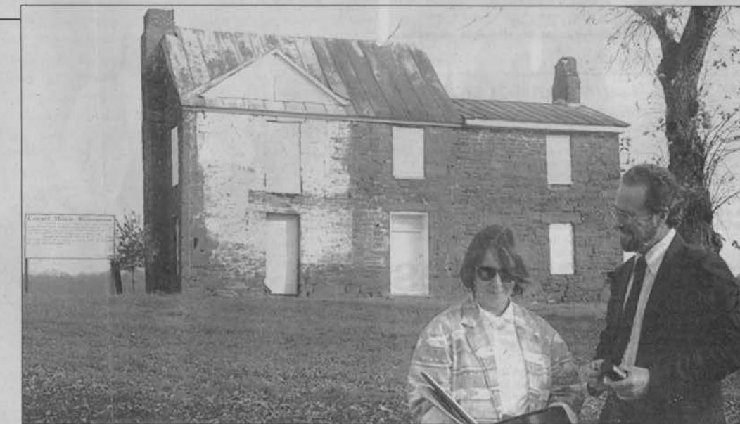
Rebecca L. Stevens, regional historical architect, left, prepares to tour the Conner House with William A. Malcom, director of Parks and Recreation for the city of Manassas Park. Stevens was invited to tour the site of the historic mansion to make recommendations on how funds can be obtained to restore the structure. (Bennie Scarton Jr., Journal Messenger.)
