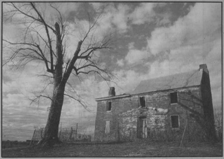
The Conner House, which once served as a Civil War hospital, is slated for restoration.
