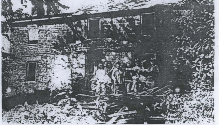
Saving the Building A group of women from the Manassas Park Woman's Club and Explorer Post 1371 were out in full force Saturday to help clean up the property around the Conner house in an effort to save the historic building from being torn down. Tossing aside a beam from the old porch are from the left, Claire Graver, Donna Murphy, Kitty Gunter, Myra Kittrell, Tina Reed, Robert Graver, Gladys Reed and Delinda Hinnant.
