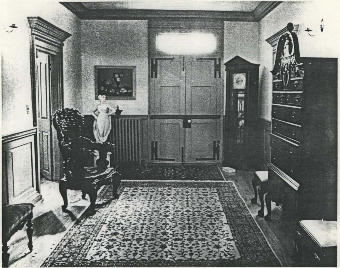
Front hallway at Effingham, showing a perfect example of "H" hinges. Paneling and doors are original; floors and plaster are new
