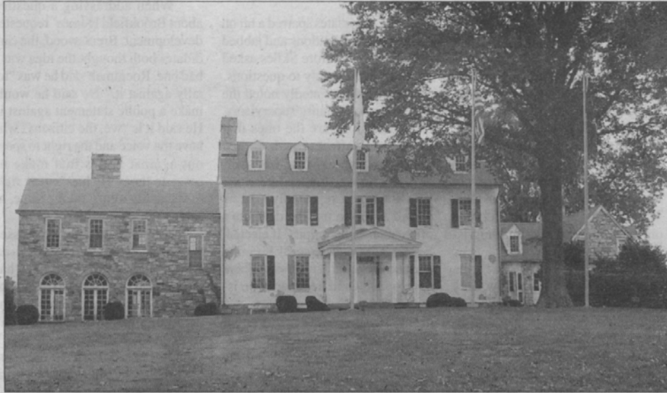
Preservation process planned for this manor house.
