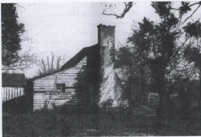
The oldest house in Haymarket is believed to have been built by a Mr. Barnett, a shoemaker, in 1800. It is a log cabin covered with clapboard.
