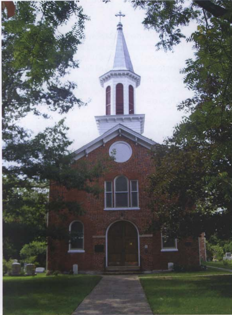
St. Paul's Episcopal Church, consecrated in 1833, was completed in 1803 as the Superior District Courthouse, serving Prince William, Fauquier, Fairfax and Loudoun counties.
