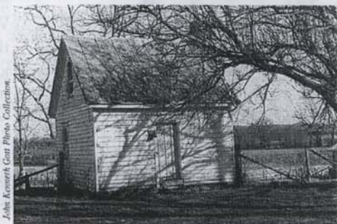
One-and-a-half story quarters at "Hazelwood", 1979.
