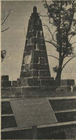
VANDALIZED —Shells like the one atop this monument were stolen.
