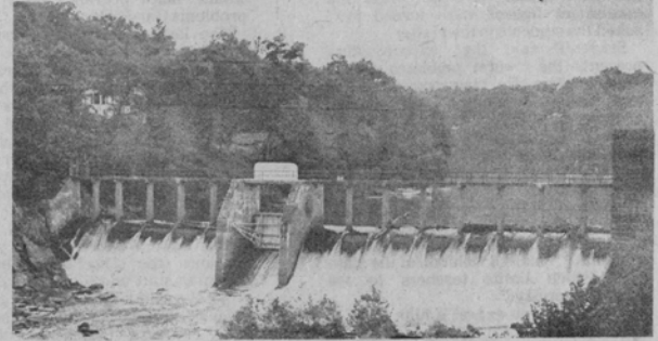
The Lake Jackson Dam constructed in the late 1920s by C.W. Alpaugh and later completed by the state.
