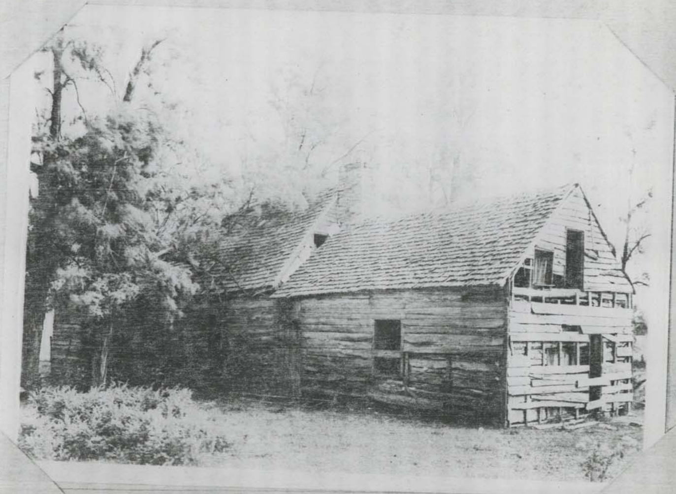
Historic American Buildings Survey John O. Brostrup
