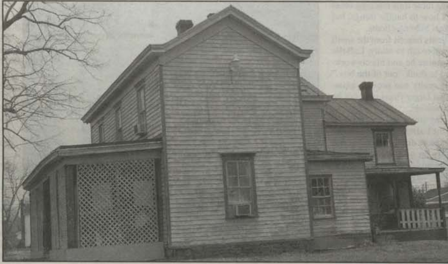
Union Col. Hutchins' house stands as originally built in 1895 except for porch lattice at 6706 Jefferson St. for which a builder has submitted a permit for demolition.
