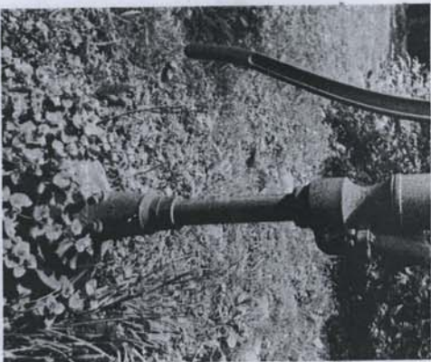
Hand pump has been replaced by indoor plumbing
