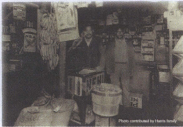
OGLE HARRIS & SONS GENERAL STORE ON WASHINGTON STREET, CIRCA 1940. OGLE AND SON ARTHUR IN PHOTO. Photo contributed by Harris family.
