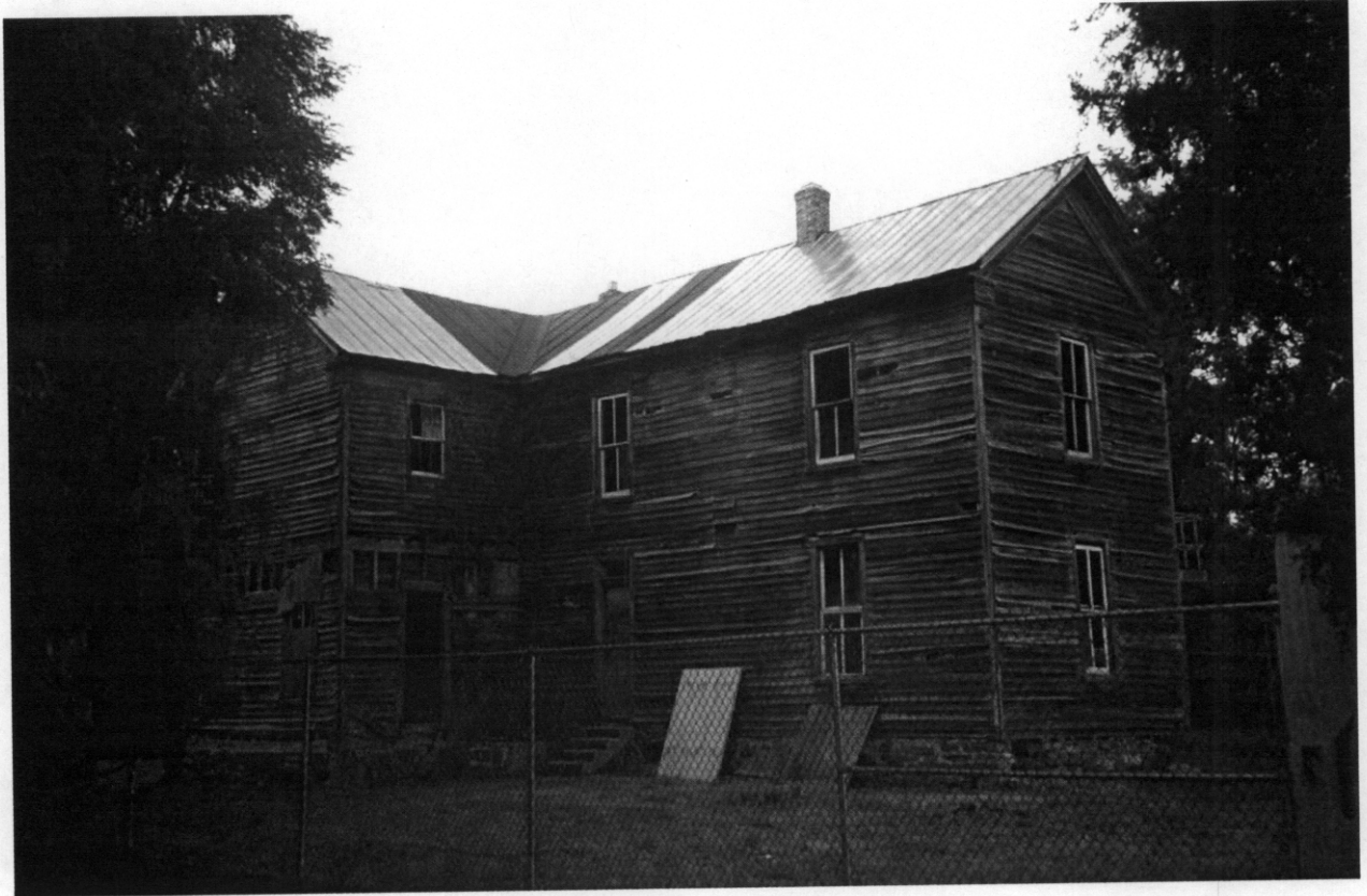
Brawner House, West and South Elevations, 2002
