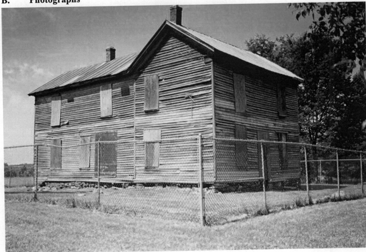
Brawner House, East and North Elevations, 2004
