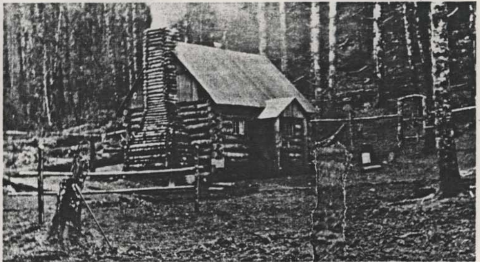
Grace Bear's home in the forest. The log chimney frequently had to be relined with mud. (Photo courtesy James C. Fulton)
