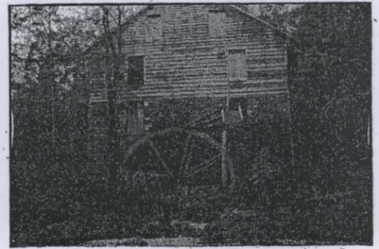
Old mill on Quantico Creek, at Dumfries, Va., once turned by flow of the stream, since silted up.
