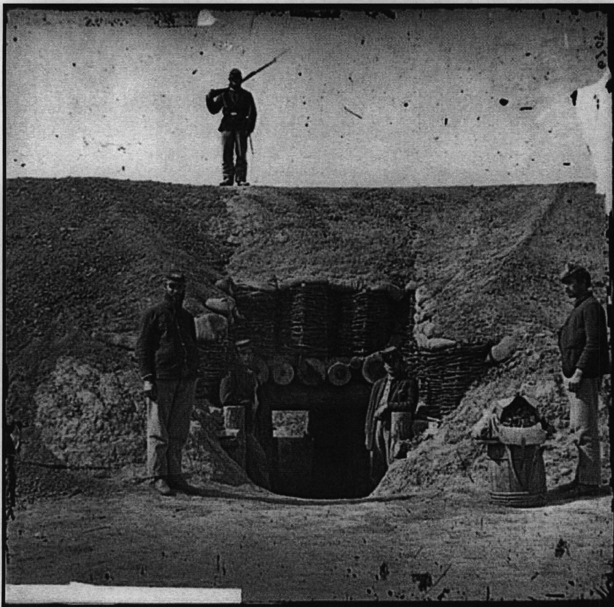
Figure 31 - A bombproof magazine, as would have been installed at the Shipping Point batteries 128
