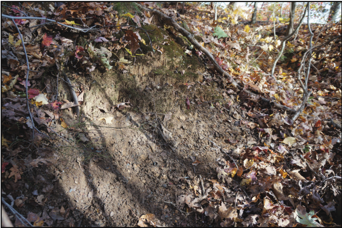
Figure 6-4: Detail of Typical Erosion Seen on Earthworks - Facing North
