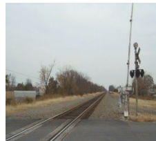
Existing Railroad Right of Way
