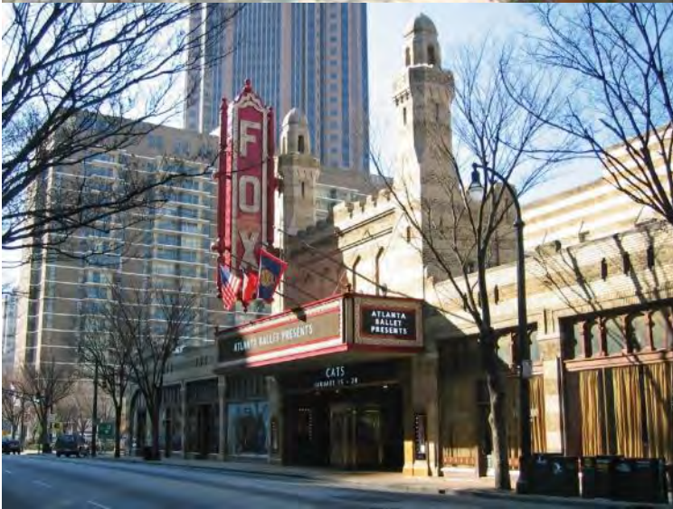
Primary building entry oriented towards street
