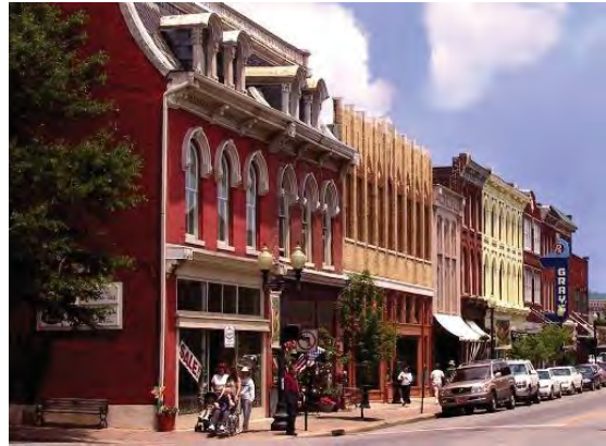
Vertical articulation of buildings
